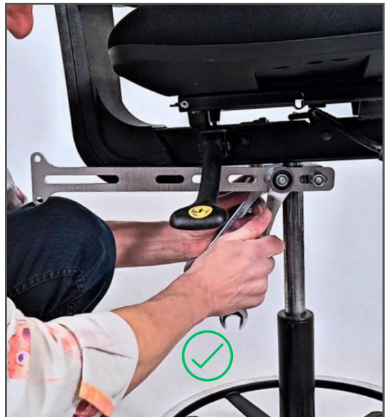
Image 12. Adjust with the bracket at a slight incline.
